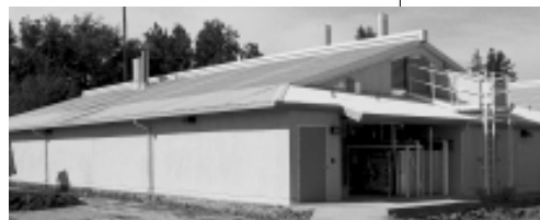
JAX® West Facility on U.C. Davis Campus
